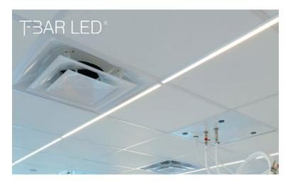
T-BAR LED becomes a structural part of the ceiling system by replacing cross tees.
