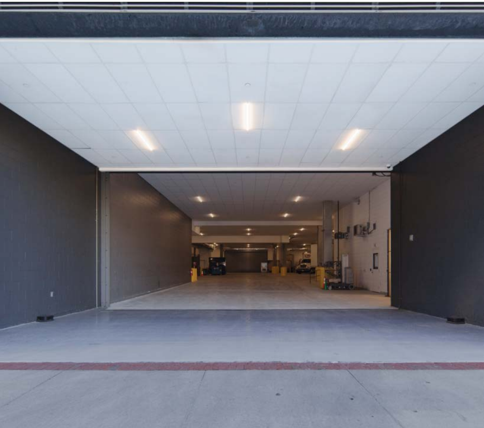
Van Ness Building – Boston, MA Samuels & Associates
